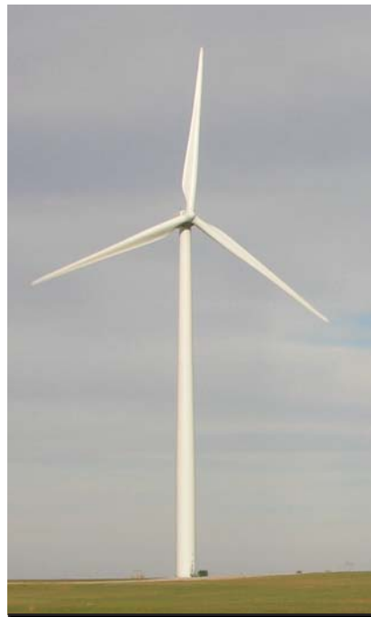
A Weatherford Wind Energy Center Turbine in perspective. Photo by Stephanie Buway
